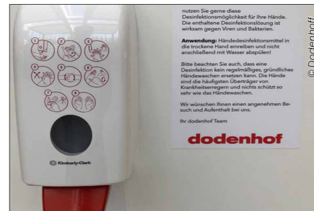
Hand disinfection in sanitary areas
