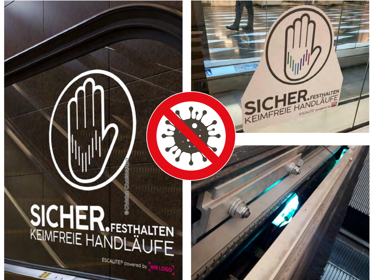
↑ Installation of an innovative UV technology: Germ-free handrails through physical disinfection of hand-held and contact points (in the escalator area)
