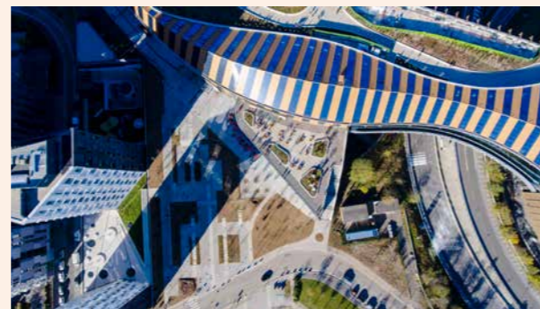
Merlata Bloom Milano is intended to be nothing less than the vibrant heart of one of the largest mixed-use areas in the first Urban Smart District of Milan, Italy.
