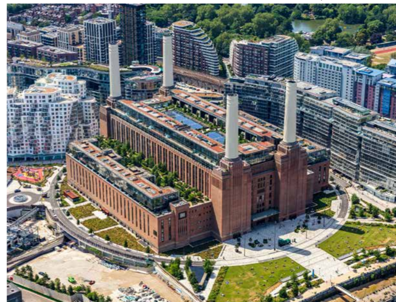
IMAGES: BATTERSEA POWER STATION / HIGH LEVEL PHOTOGRAPHY
