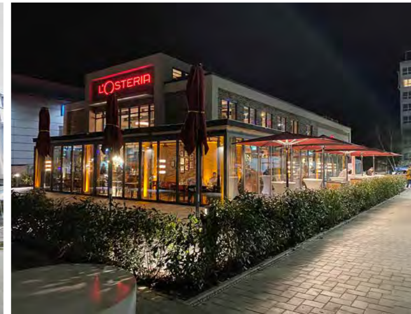
The refurbishment of parts of the Rhein Neckar Zentrum is complete and was officially opened (left). Among other things, a freestanding L'Osteria restaurant has been opened in the former DIY store parking lot (right).
